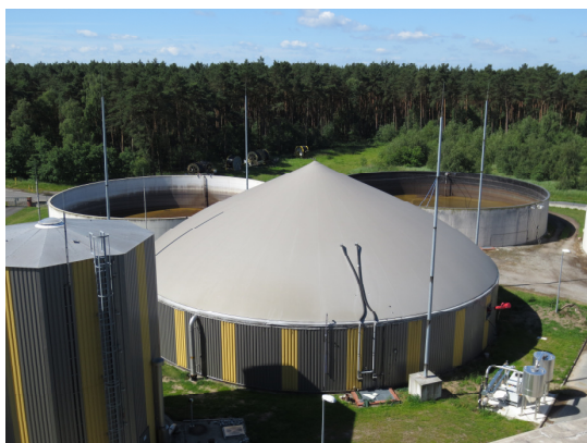
Biogas plant in Germany
